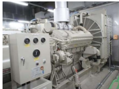
Emergency power supply equipment
