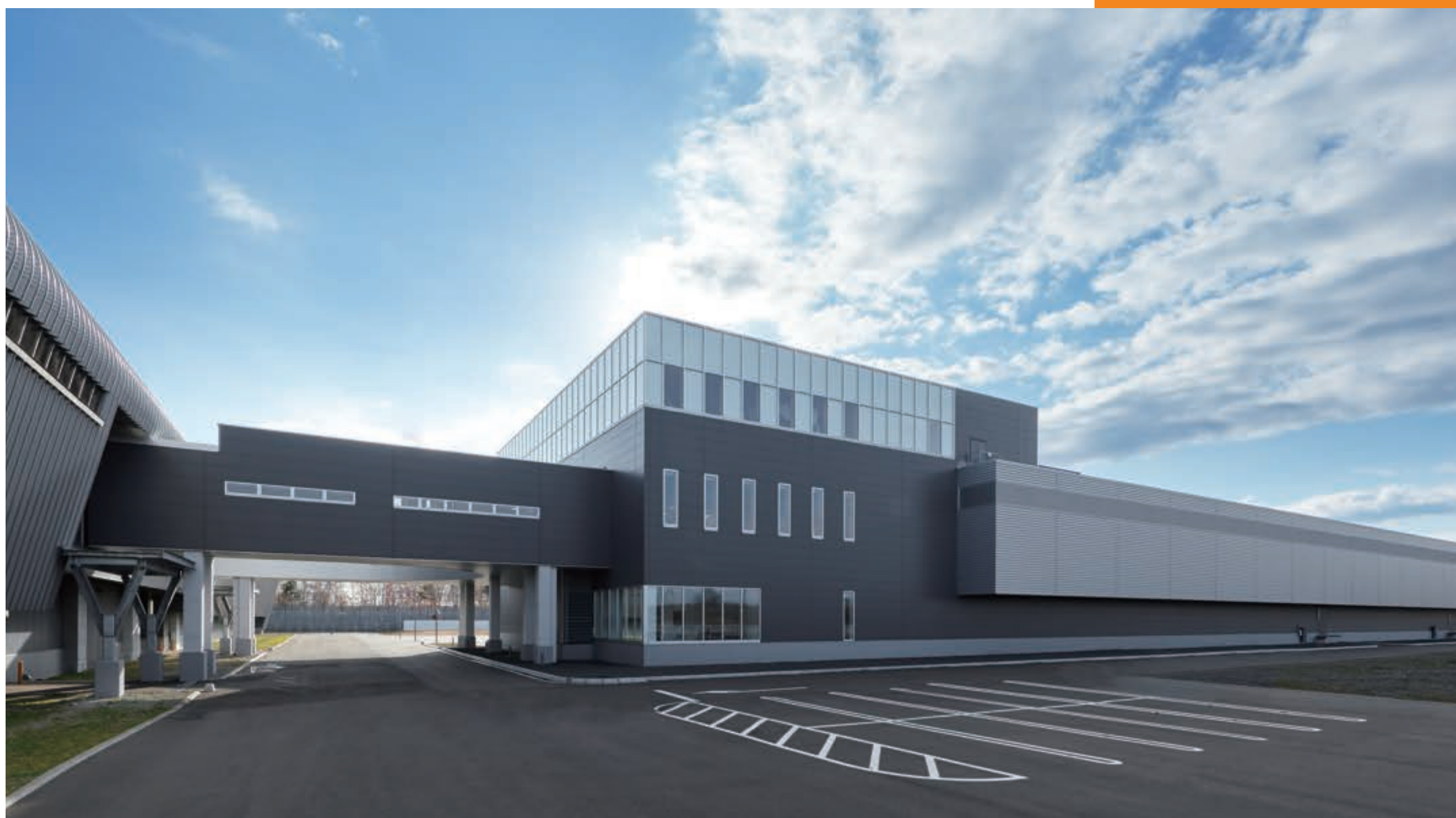
▲ Ishikari Data Center Building No. 3
