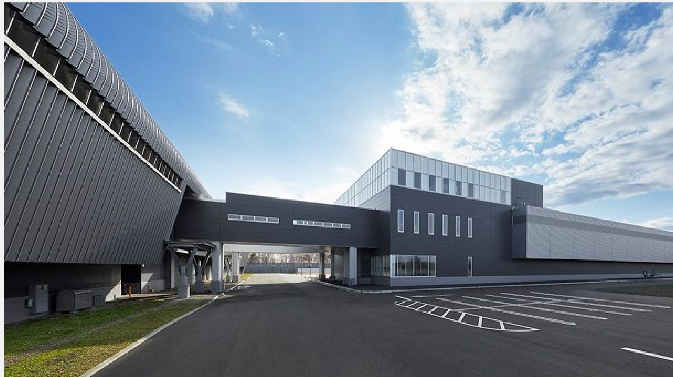
Appearance of Ishikari Data Center (front: Buildings 3, left: Buildings 1 and 2)
